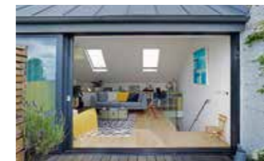
ANOTHER LEVEL Ursula and Alex built an upper-floor level on top of their existing flat roof townhouse, and this was then given an attractive pitched zinc roof. Building upwards was an inspired idea, as the family now have a large, light-filled sitting room, which leads out onto a stylish and spacious new roof terrace.
